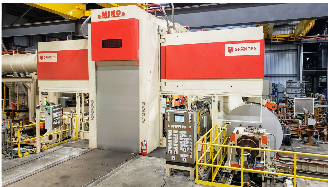
New cold rolling mill at Gränges' plant in Huntingdon, Tennessee.
